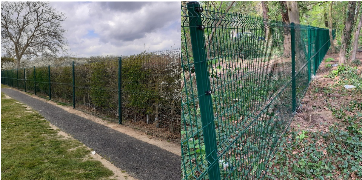
Figure 1: Examples of proposed 1.5m high welded mesh fence boundary treatment along eastern site boundary.
